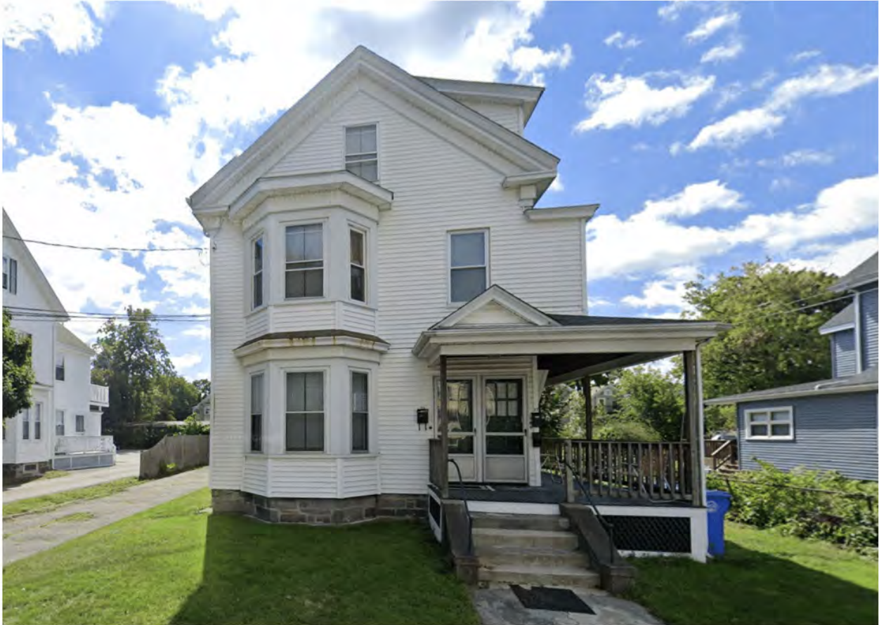
79 Cherry St. is in a neighborhood with historic homes. Image from Google Street View.
