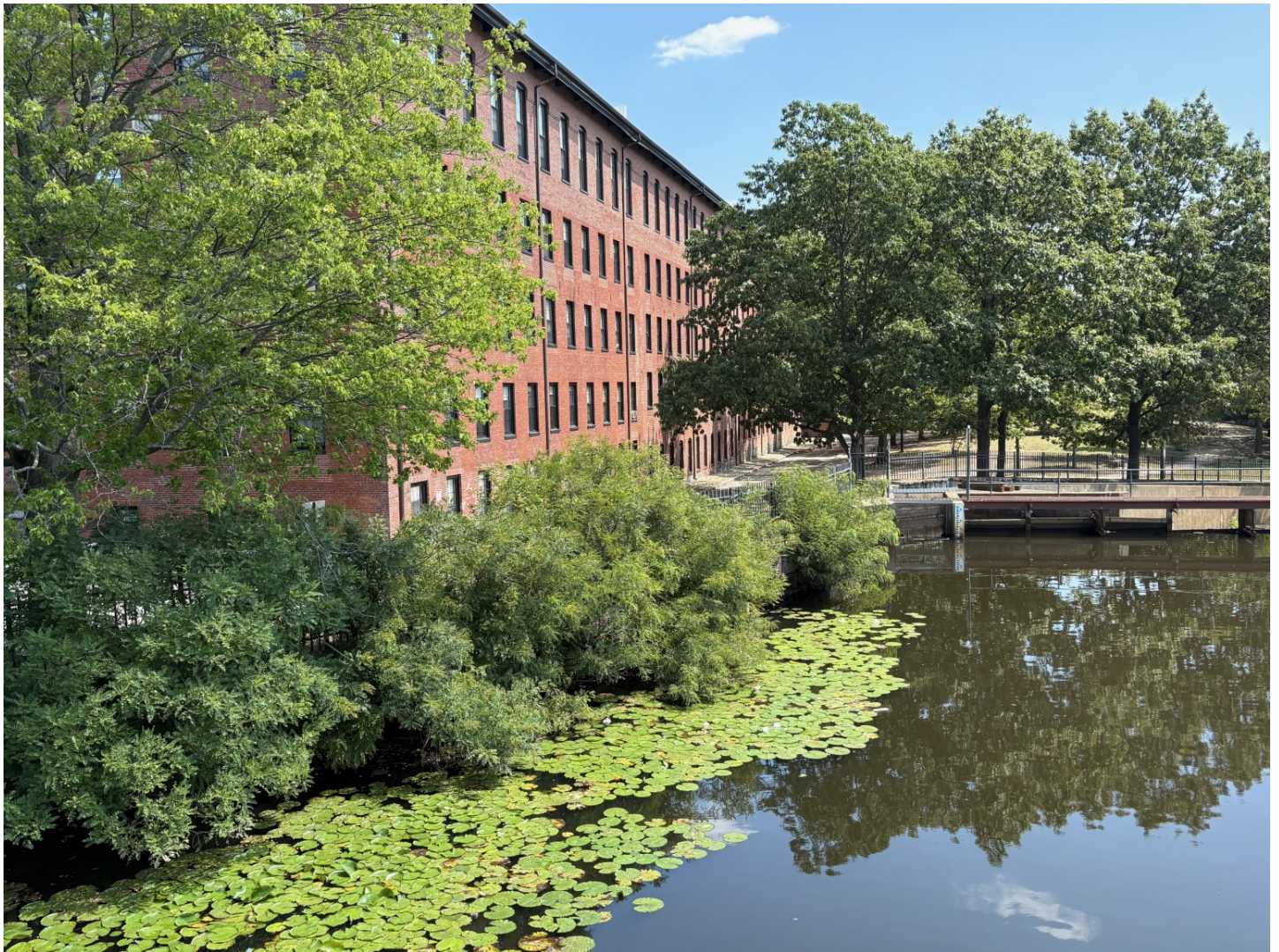
Cabot Mills by the Charles River dam.
