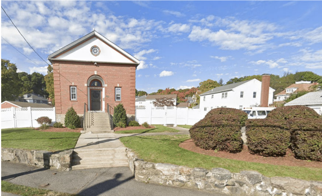
Opportunities for Inclusion building at 15 Fiske Ave. Photo from Google Street Image.
