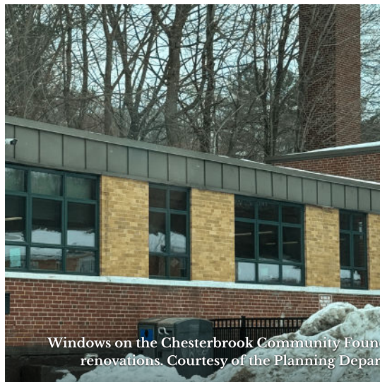
Windows on the Chesterbrook Community Foundation before renovations. Courtesy of the Planning Department.
