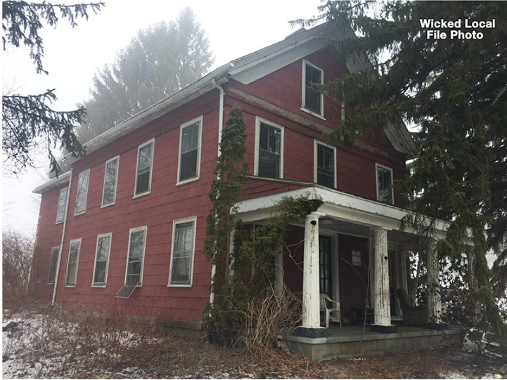
Cardinal Cottage prior to its exterior renovation.
