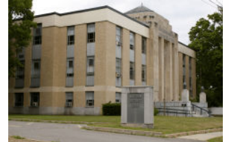
Waltham District Court.
